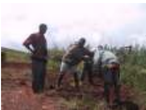
Repairing the road to Juniper Forest.
