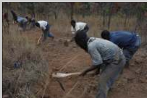
Road cutting at Lower Chelinda
